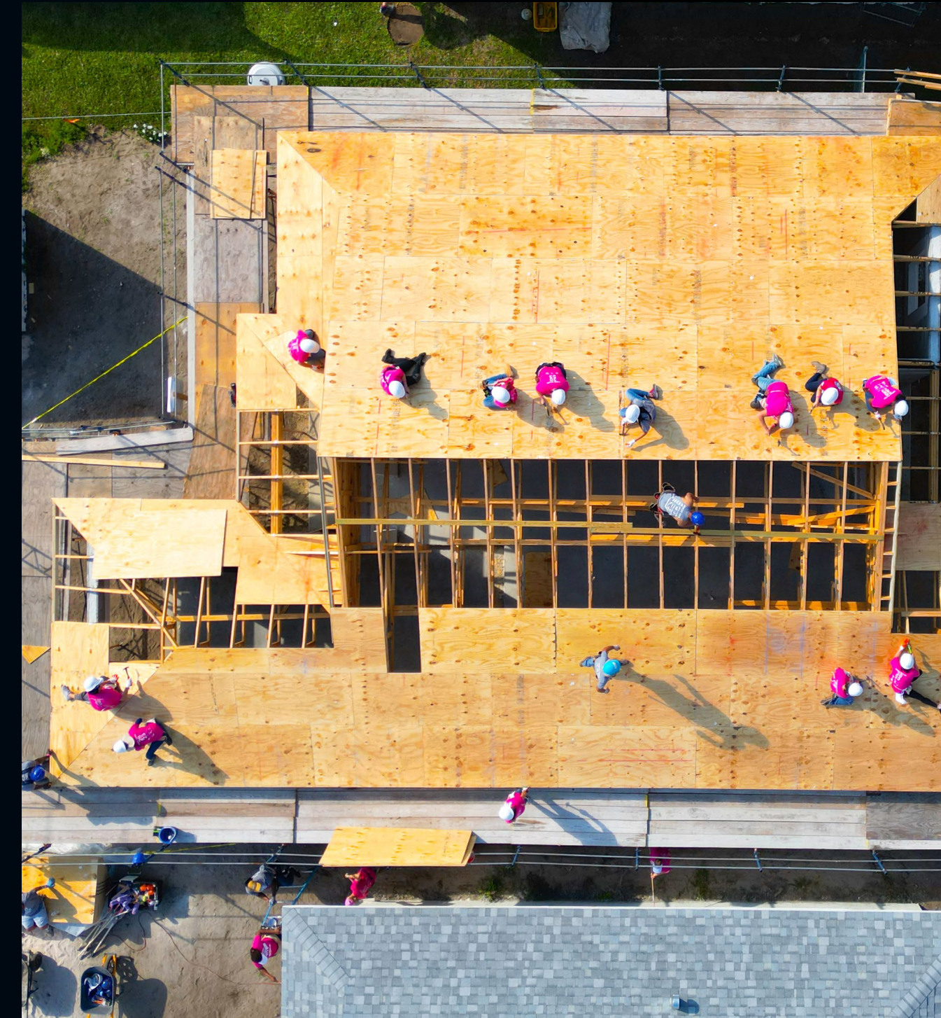
The Boca Raton Airport Authority joined a team of over 100 women for Habitat for Humanity's Women Build 2023, an initiative focused on providing affordable housing to families in need.
