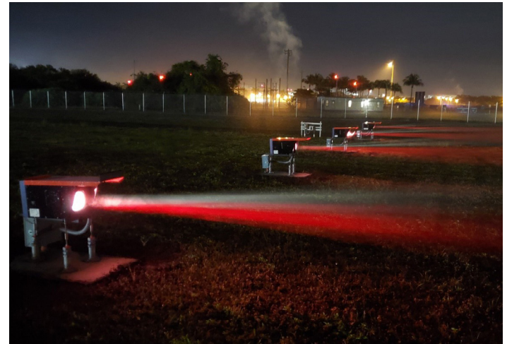
The PAPI lights will all appear red from the ground, but indicators appear red and white when viewed by the pilot on proper approach angle.
